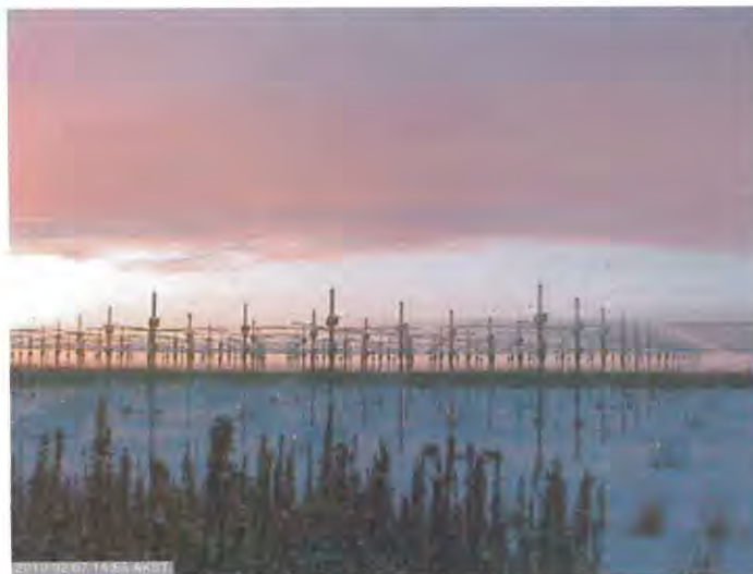
The HAARP-antenna array at Anchorage, Alaska 115
